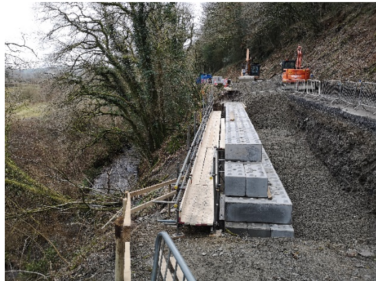
Lego land? Work in progress to repair the road
